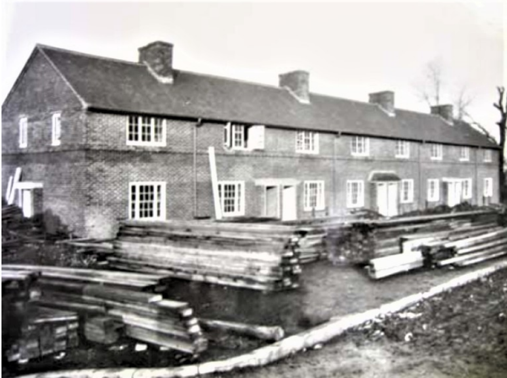
Laneway under construction
