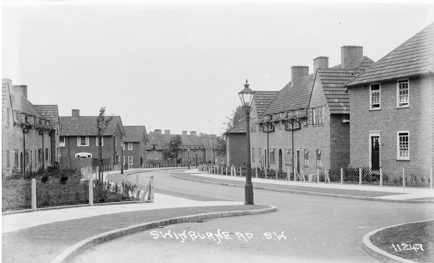
Swinburne Road just after construction – the privet hedging is very new
