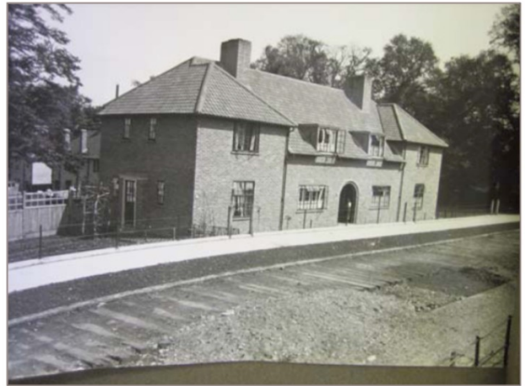
Parkstead under construction
